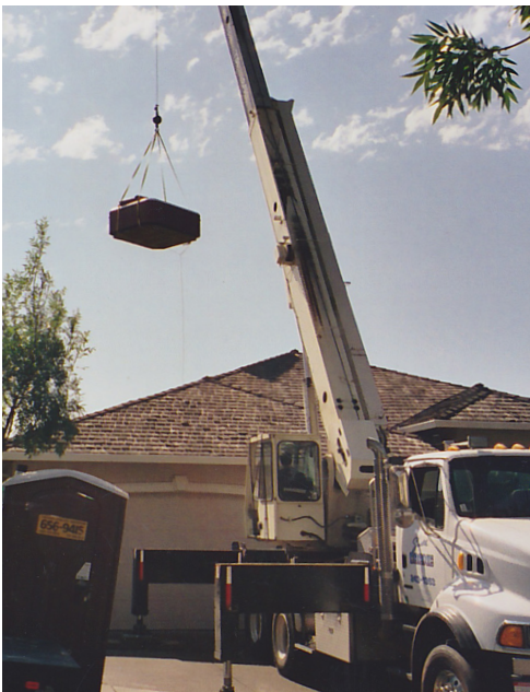
A crane to bring in the hot tub.
